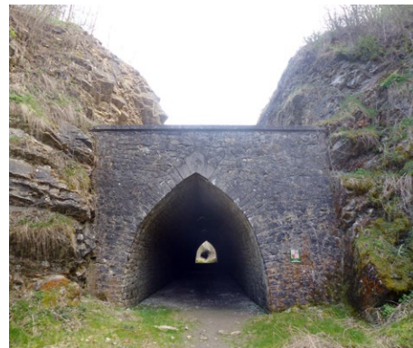
Tunel v lomu Požáry.
